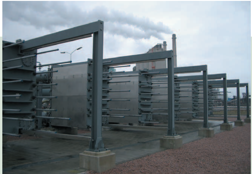
Energy center (Lyondell, Holland / UX-100, 11units)
