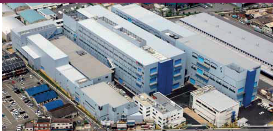
Hisaka Works, Ltd. / Konoike Plant
